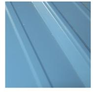
The same panel, after red rust has been removed by gently scrubbing the surface using a mild cleaner and pad
